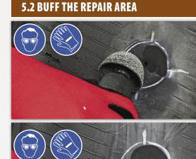
or electric buffing tool with a clean buffing rasp, 18 to 36 grit and remove all vent lines until you get a completely smooth surface. Continue lightly buffing the repair area to a smooth velvety finish (RMA Buff Texture 1 or 2) by putting slight pressure on the buffing tool and keeping it in constant movement.
